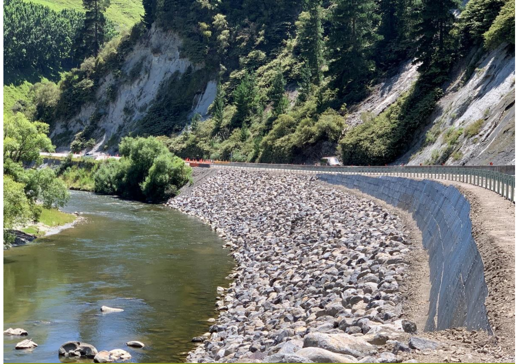
Hapokopoko Riprap & MSE wall (SH4)
